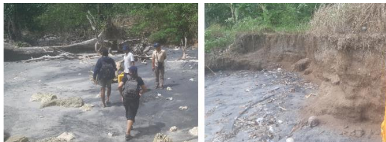
Fig. 3. Documentation of erosion during site visit
