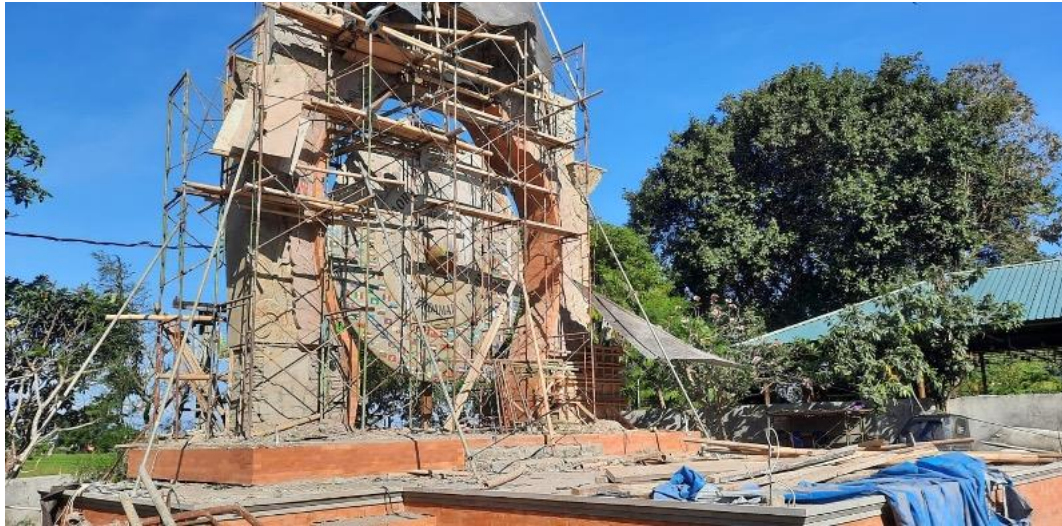
Picture 2. Location of the World Peace Gong under construction in Kertalangu Cultural Village
